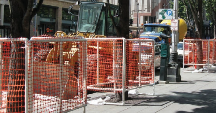
Figure 3: Tree Protection Fencing (Credit: City of Seattle)
