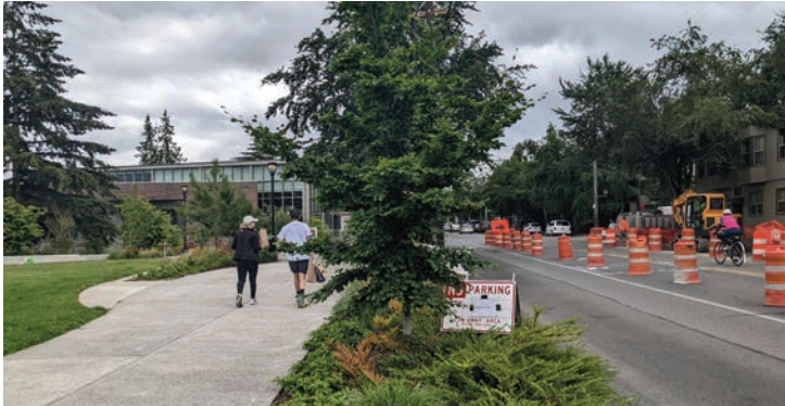
Figure 5: Open Tree Trench with Step Out Zone (Credit: Toole Design)
