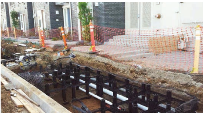
Figure 6: Installation of Soil Cells at Back of Curb (Credit: DeepRoot)
